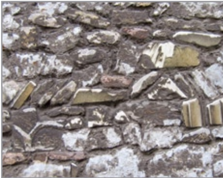
The east wall at St Mary's, Bedford is a hotch-potch of different stones, tiles and re-used building materials.
