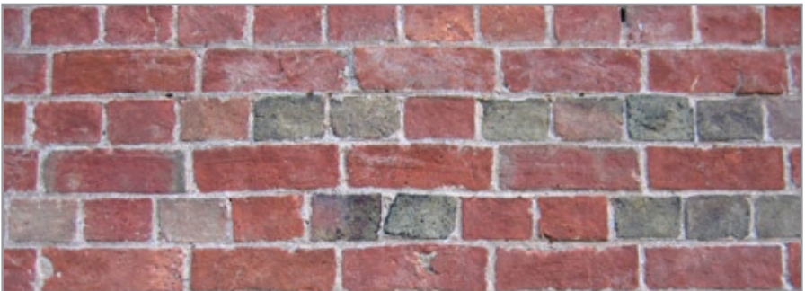
An early 1800s Bedfordshire house wall built in ‘English Bond’. Bricks can be laid in many patterns.
