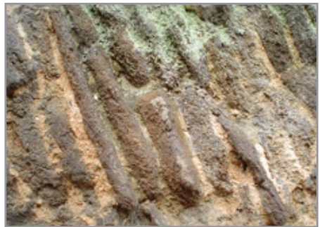
Above: a wall at Potton typical of many on the Lower Greensand outcrops. Slabs of red-brown sandstone are held together with mortar.
