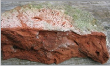
A fragment of Roman brick with a layer of Roman mortar (made with fragments of brick instead of aggregate) on the upper surface.
