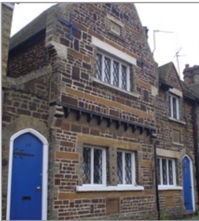
Above: larger blocks of sandstone have been used to build Wilkes Almshouses in Leighton Buzzard. The quartz cementing the sands produces a very strong stone, darker in colour than the iron oxide alone.
