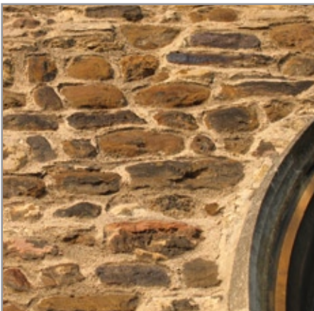
Left, local sandstone from the Lower Greensand.
