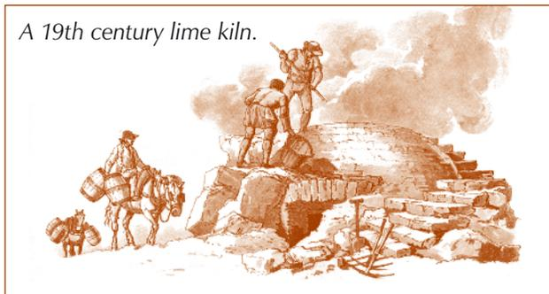
and some oxygen to leave calcium oxide, known as *quicklime*. This is added to water<sup>1</sup> in the process known as *slaking*; *lime* is the product of the resulting violent reaction. Relatively little water yields powdery hydrated lime; more water creates lime putty (the basis for lime mortar) and eventually limewash. These lime products are *non-hydraulic*, which means they harden by drying, or by reacting very slowly with atmospheric CO<sub>2</sub>.
